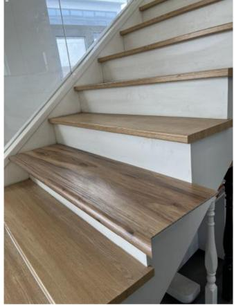
5. Seal the edges with glue on the sides.
