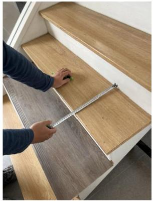
2. Measure the appropriate size for the Stair Tread and then cut it using a table saw/circular saw.
